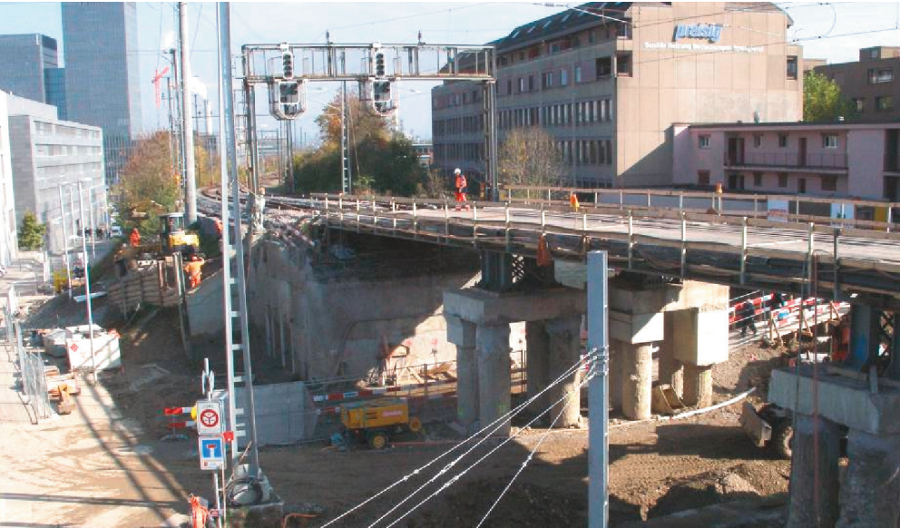
Reconstruction of the 100 year old railway bridge carrying two railtracks.
