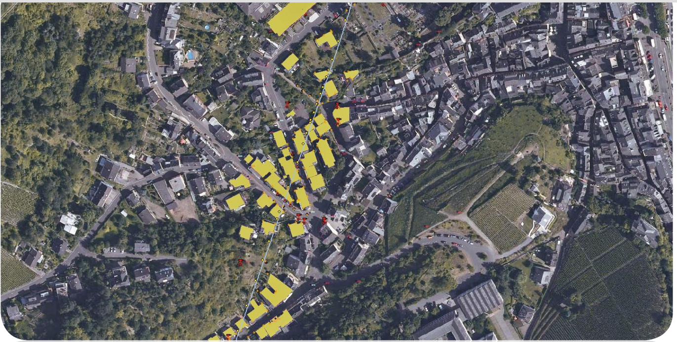
■ The tunnel crosses under numerous houses in Cochem, some a mere three meters above.
