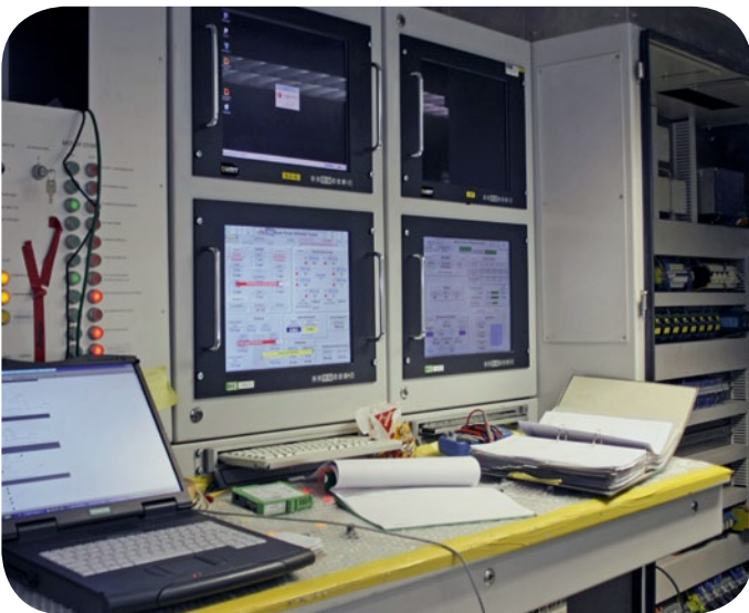
■ Current measurements at the TBM control center.
