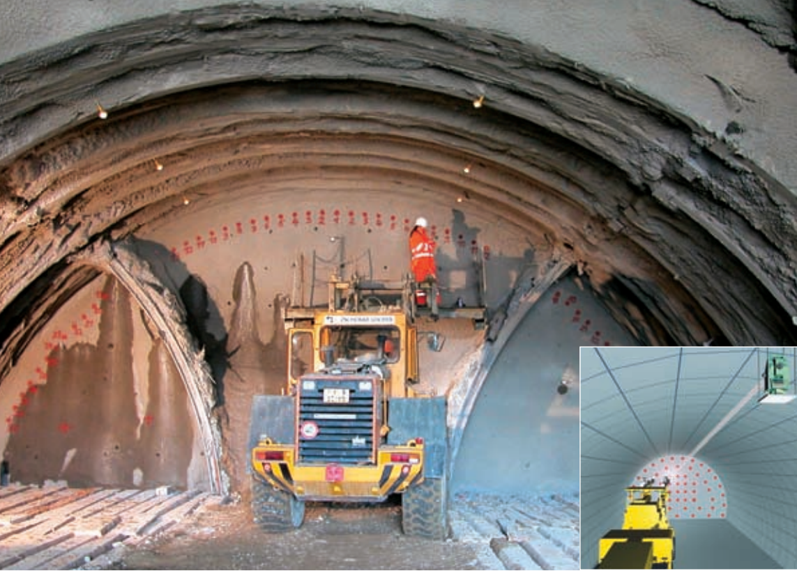
Drill and blast (BLAST) Automatic, manual or timer controlled display of blast pattern
