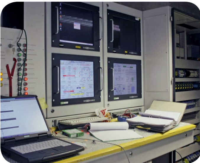
■ Current measurements at the TBM control center.
