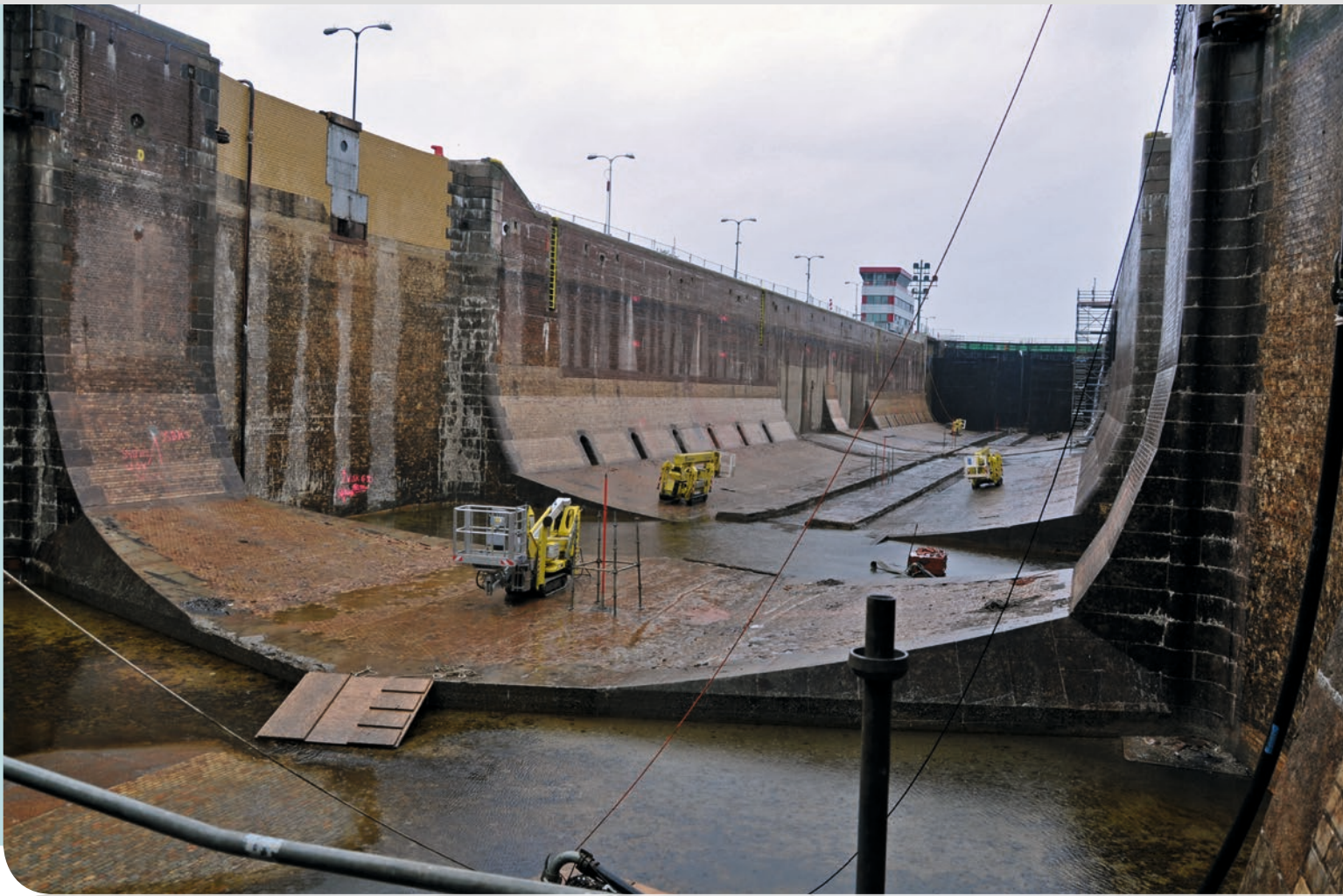
■ Ready for safe renovation: The empty ship lock gets inspected while the structure is being monitored.
